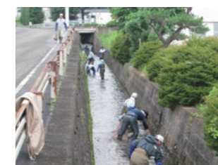
Volunteer river cleanup work in the Sakura area
